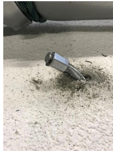
Photo 5 – Specimen after testing
